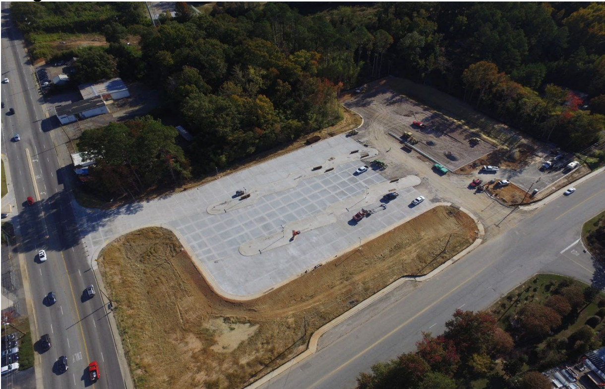
Aerial view of the Lucius Road Superstop Project.
