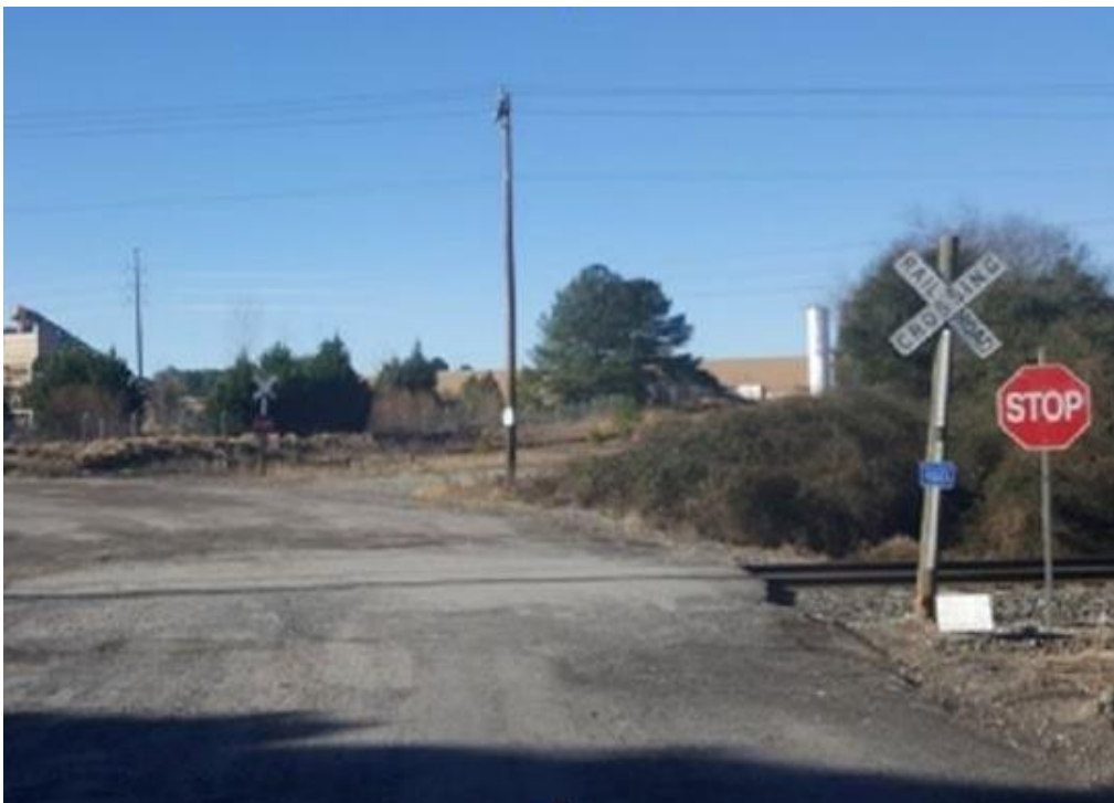
Hobart Road Railroad Crossings
